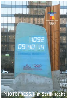
PHOTOPRESS/Kim Stalknecht Rockingham Engineering designed the internal structural steel framework behind the glass clock and wood tower as well as the concrete base.
